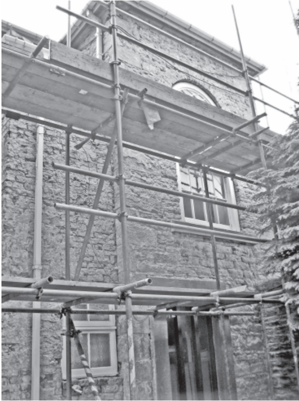
One of Lanchester's oldest buildings is ringed with scaffolding. The Lodge, part of which dates back to 1596, has thick stone walls which at some point were rendered, possibly by a Mr Ornsby in the 18th century. As part of the improvements put in hand by Dr Brunt, this rendering is being removed. It is yet to be decided if any or part of it should be replaced, but it offers the opportunity to see the Lodge as it probably was before the 18th century improvements.
