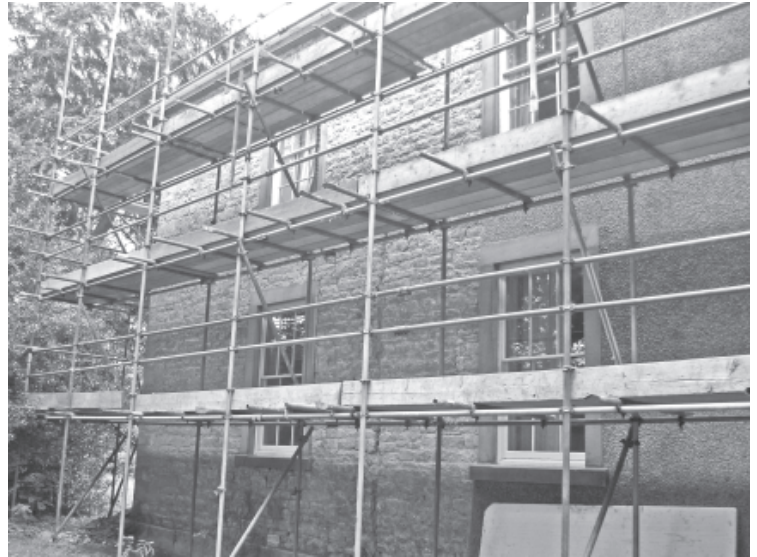
One of Lanchester's oldest buildings is ringed with scaffolding. The Lodge, part of which dates back to 1596, has thick stone walls which at some point were rendered, possibly by a Mr Ornsby in the 18th century. As part of the improvements put in hand by Dr Brunt, this rendering is being removed. It is yet to be decided if any or part of it should be replaced, but it offers the opportunity to see the Lodge as it probably was before the 18th century improvements.
