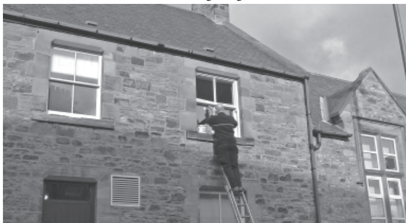
The installation of the new windows
