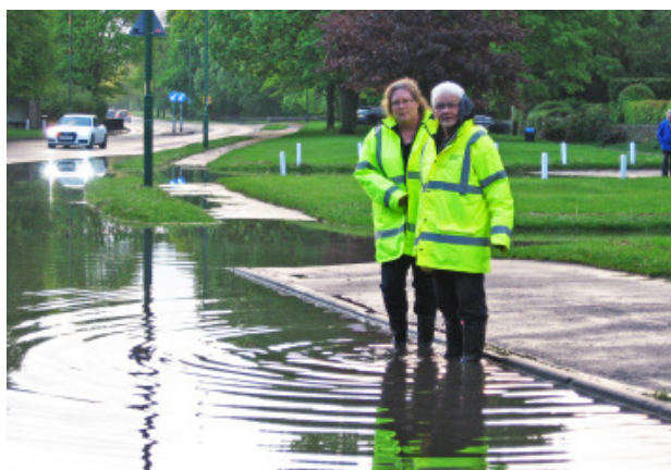
Flooding outside All Saints' Parish Church after a short deluge on 20th May. Sally Laverick and Eric Hepplewhite from the Emergency Action Group turned out to direct traffic.
